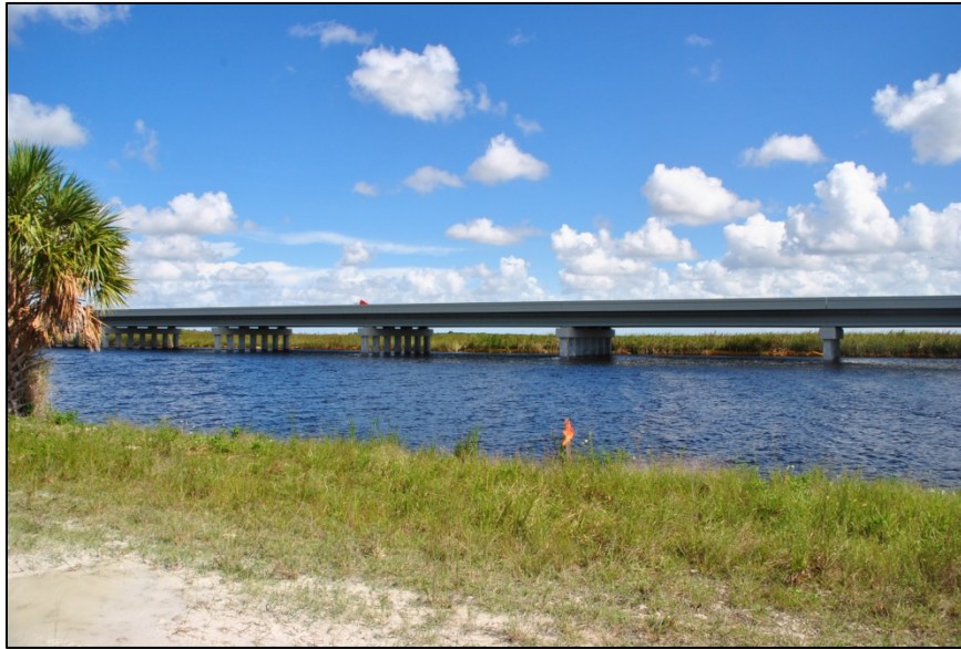
Tamiami Trail Modifications Project
