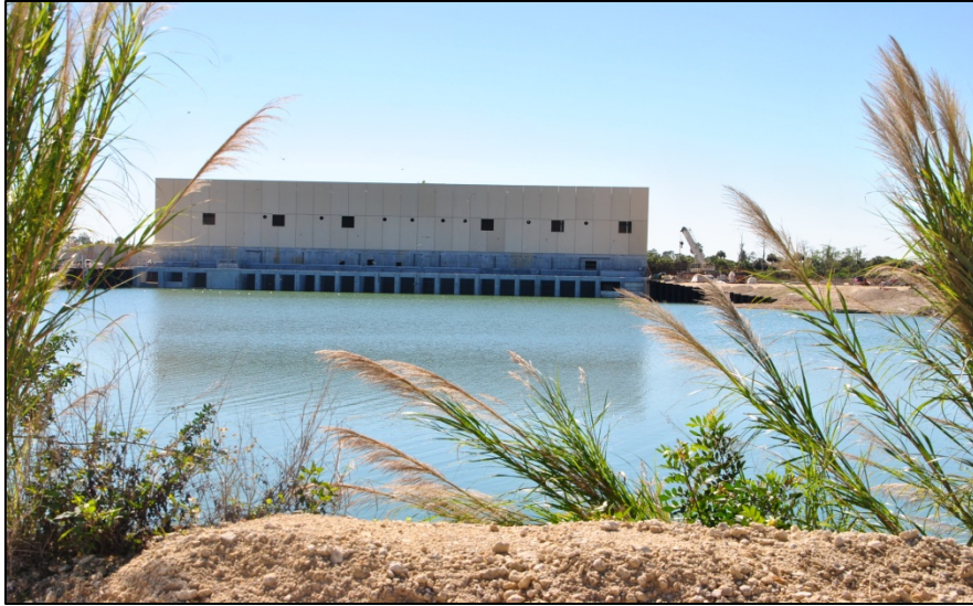
Merritt Pump Station (Picayune Strand Restoration Project)
