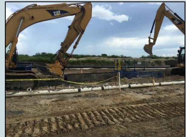
Toe trench drain test
