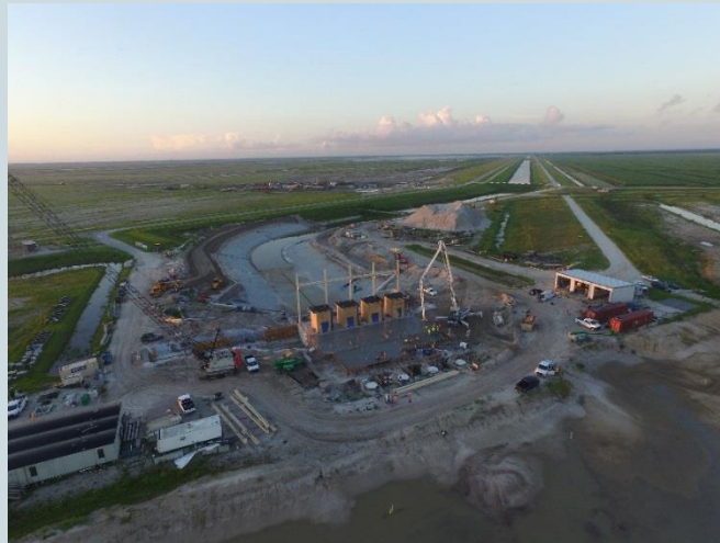
C-44 Pump Station construction 2017
