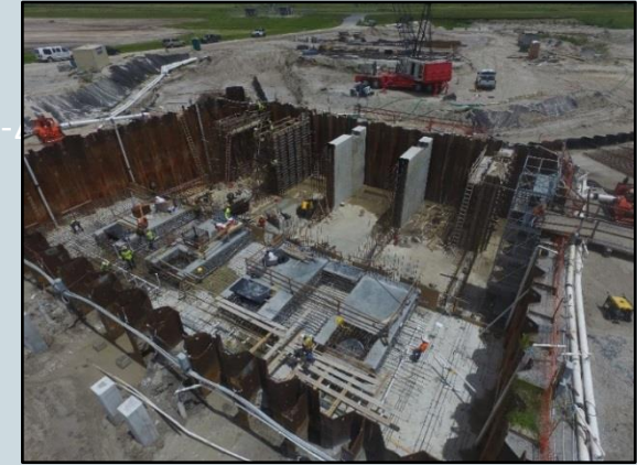
C-44 Pump Station construction aerial view 2016
