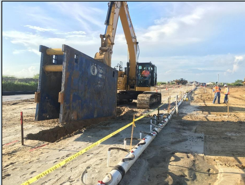
Toe trench drain test
