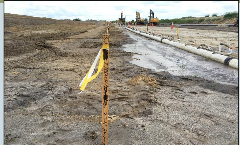
Dewatering system and survey stake
